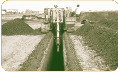
DIGGING A TRENCH TO LAY GROUND LOOPS
