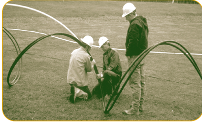
GROUND LOOP OR “SLINKY”
